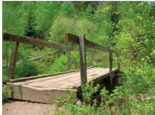
North Fork Bridge Before
