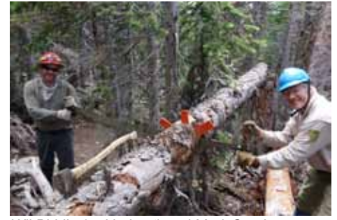
Wil Biddle (red helmet) and Mark Snyder (blue helmet) using a 2-person saw and three wedges. Thirty miles of trail were cleared.
